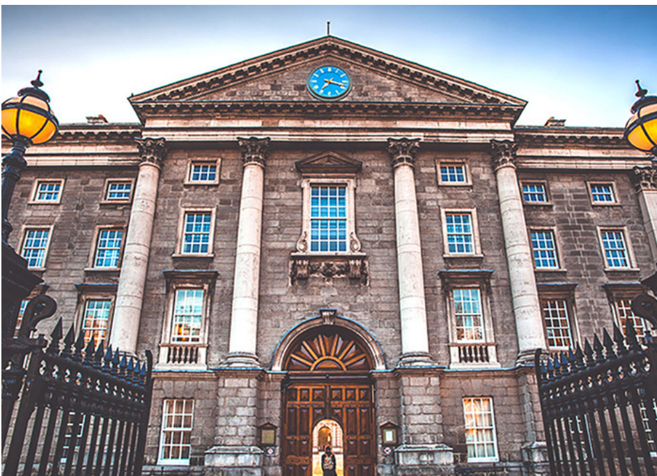
Image 1. An Ivy League college needed an update to its cogen facilities. (Images courtesy of Sundyne)
