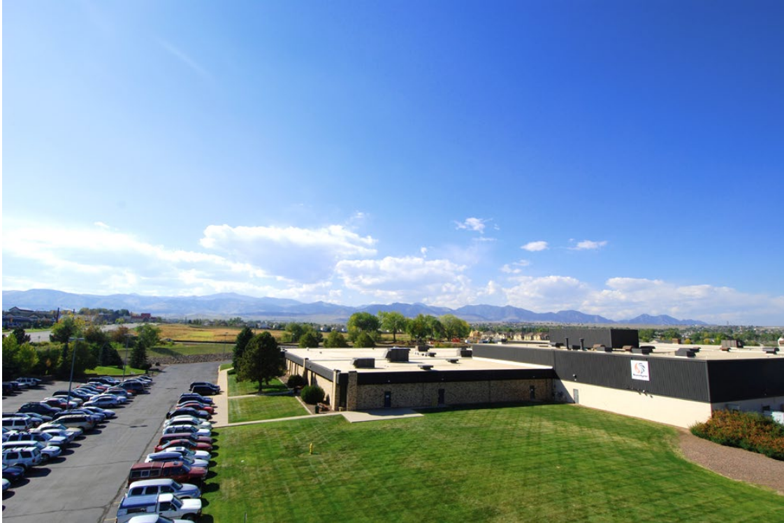
Figure 1: Sundyne Headquarters in Arvada, Colorado, USA
