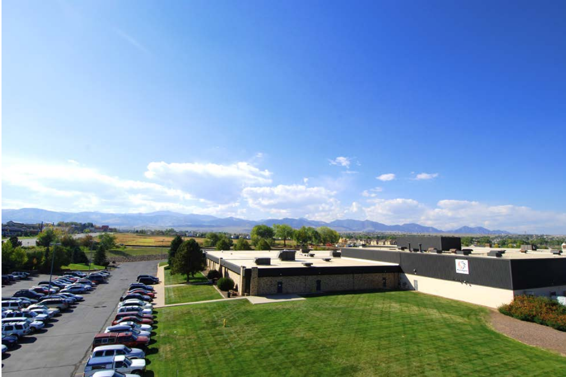
Figure 1: Sundyne Headquarters in Arvada, Colorado, USA
