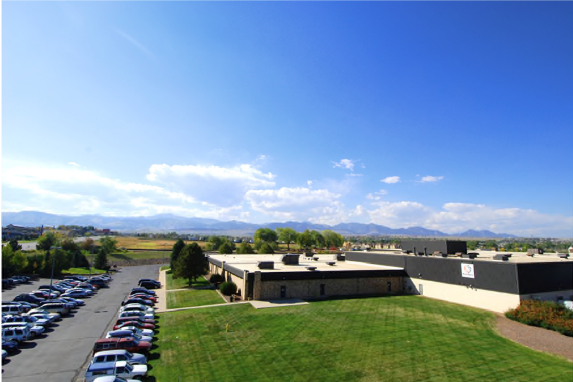
Figure 1: Sundyne Headquarters in Arvada, Colorado, USA
